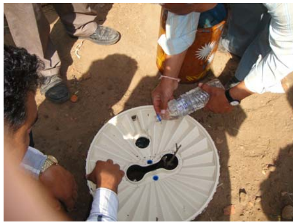
Fig.9 Adding water to prevent floating
