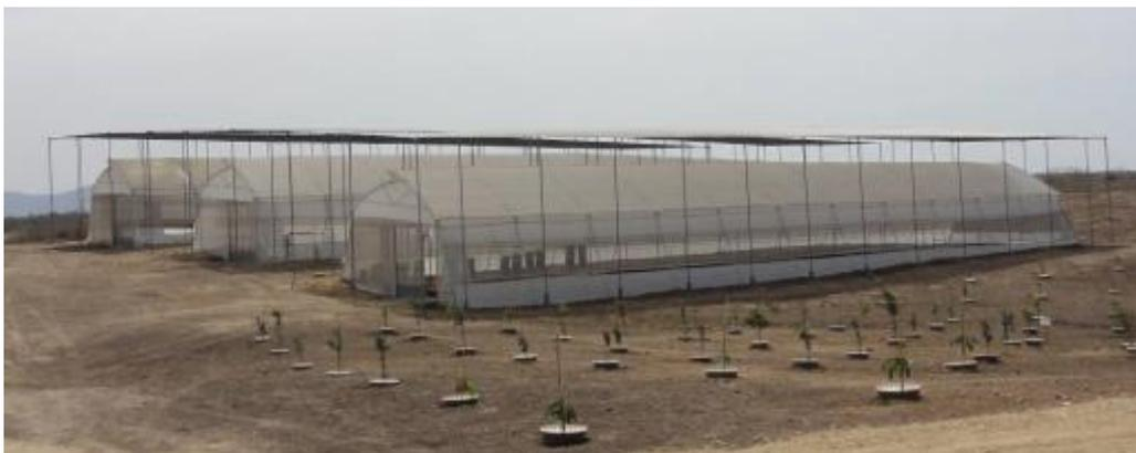
3. Use ventilation openings along the whole side. If you expect to have insect problems, add insect-screen in the ventilation openings on the side. However, in warm climates this will decrease ventilation capacity and your greenhouse may be too hot during the day.
