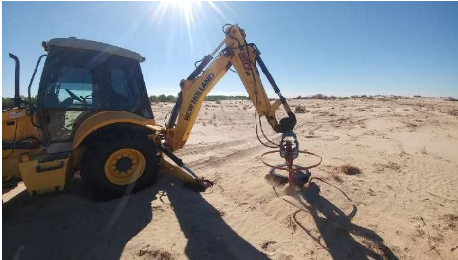
Figure 7: Excavation tests to carry out the reforestation in the determined polygons.
