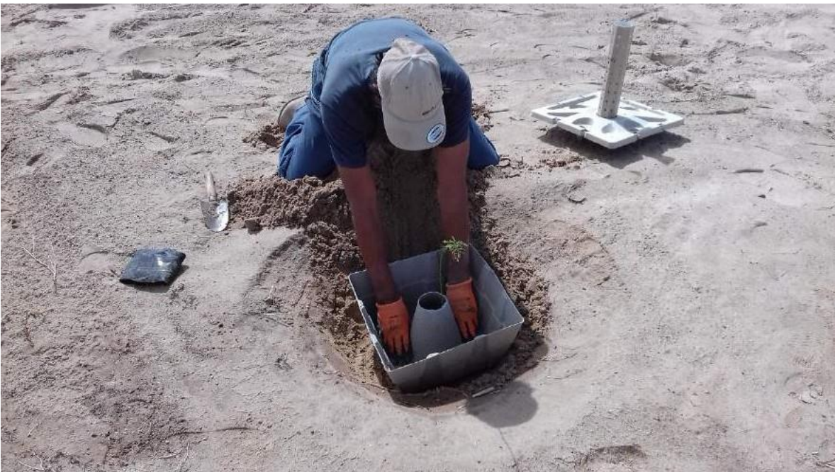
Figure 13: Installation of Growboxx ®
