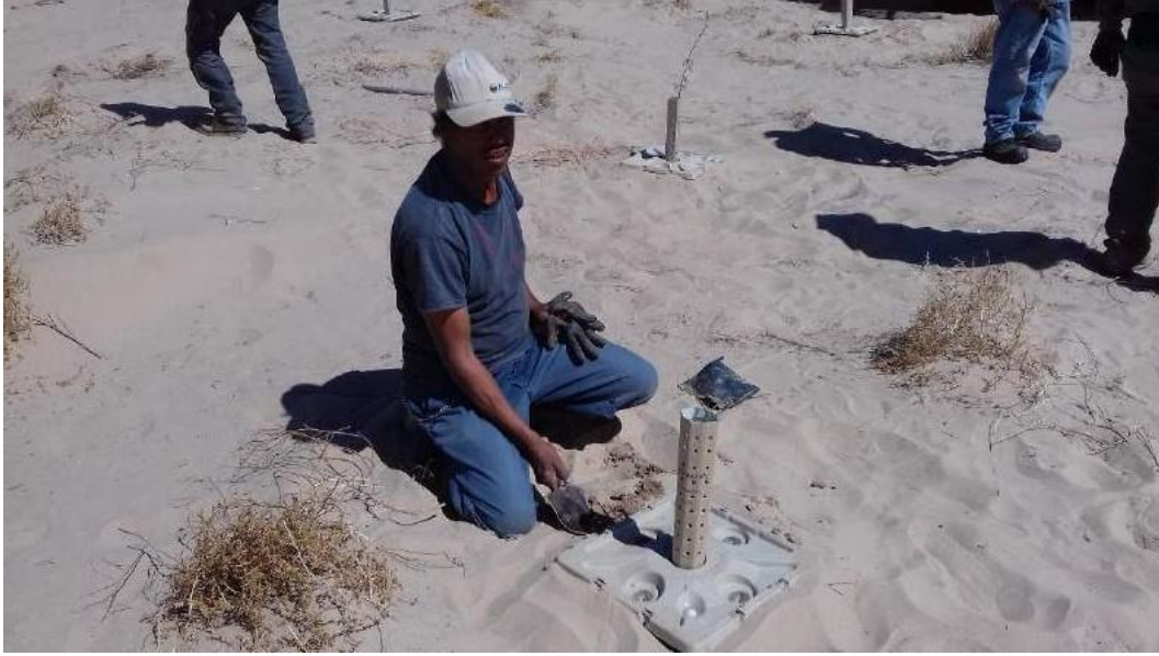
Figure 15: Completion of the Growboxx® installation
